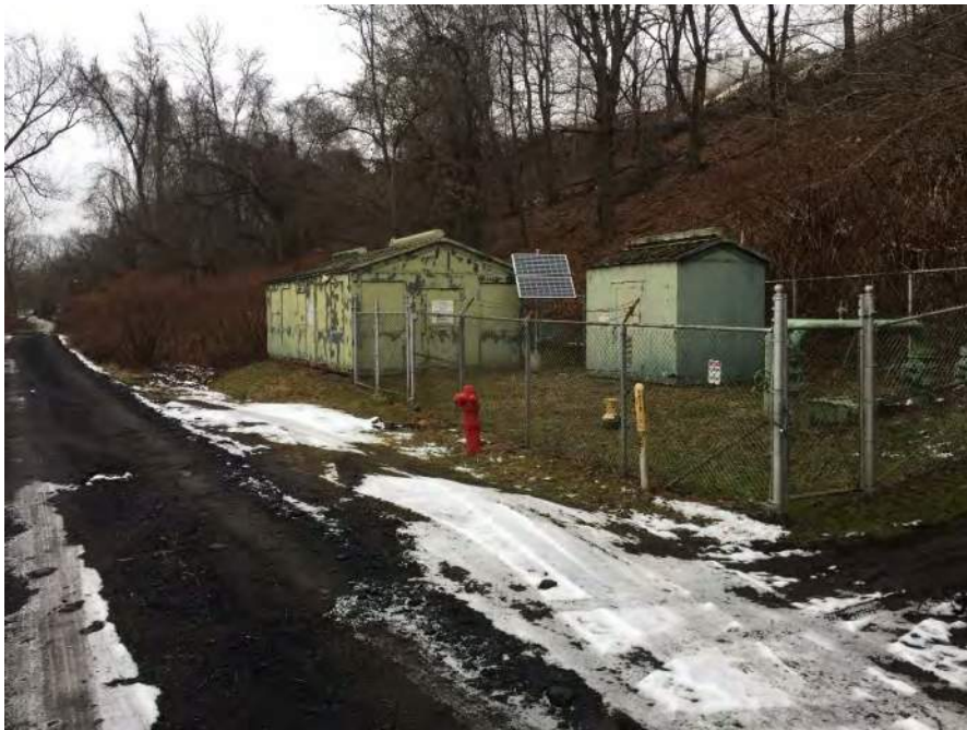
Photograph 4: Columbia Gas Transmission Station, view looking north along South Chestnut Street.
