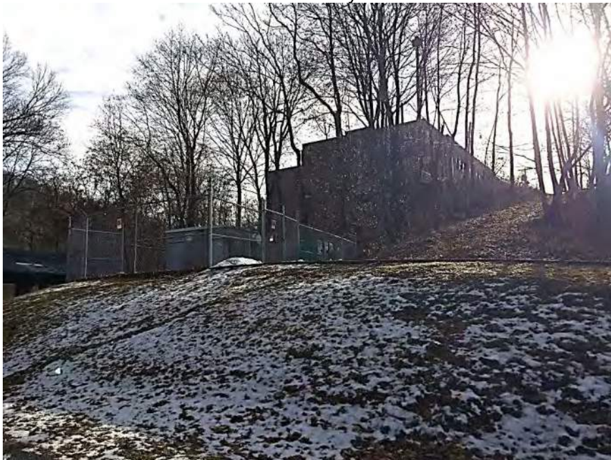
Photograph 6: View facing east showing a second municipal sewer vac station located within the New Cumberland City Park.
