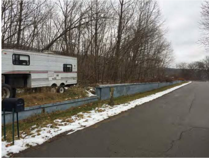
Photograph 7: View facing southeast along Pottery Road showing blue retaining wall from past land use associated with Former Pottery Mill.
