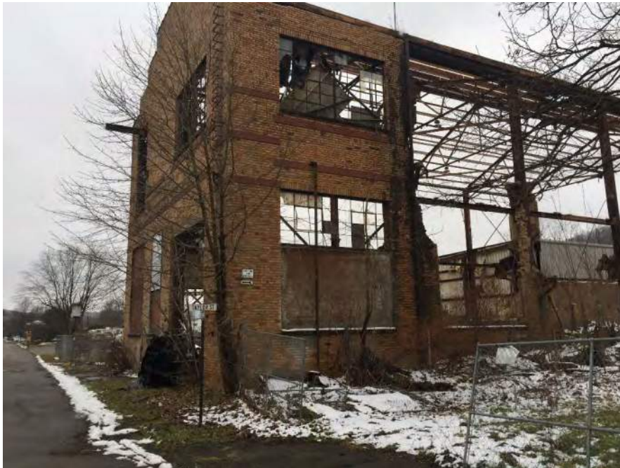
Photograph 14: View looking southwest near intersection of Taylor Street and South Chester Street at American Industrial Recycling site.
