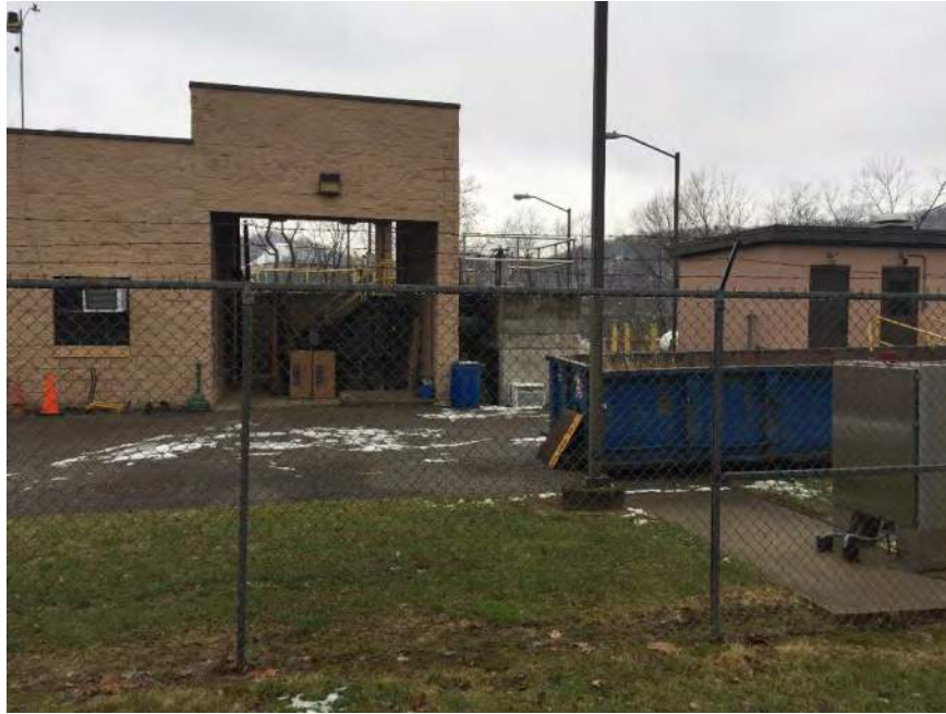
Photograph 1: Wastewater treatment plant near intersection of Industrial Park Road and WV-2, view looking west from Industrial Park Road.
