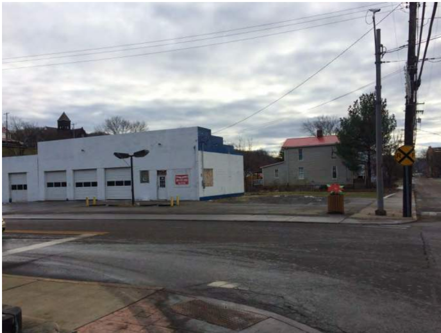
Photograph 2: View facing southeast at the intersection of North Chester and Madison Streets showing the former Bowen's Service Station. Note the filled gravel area right of the station building and dispenser area along Madison Street.
