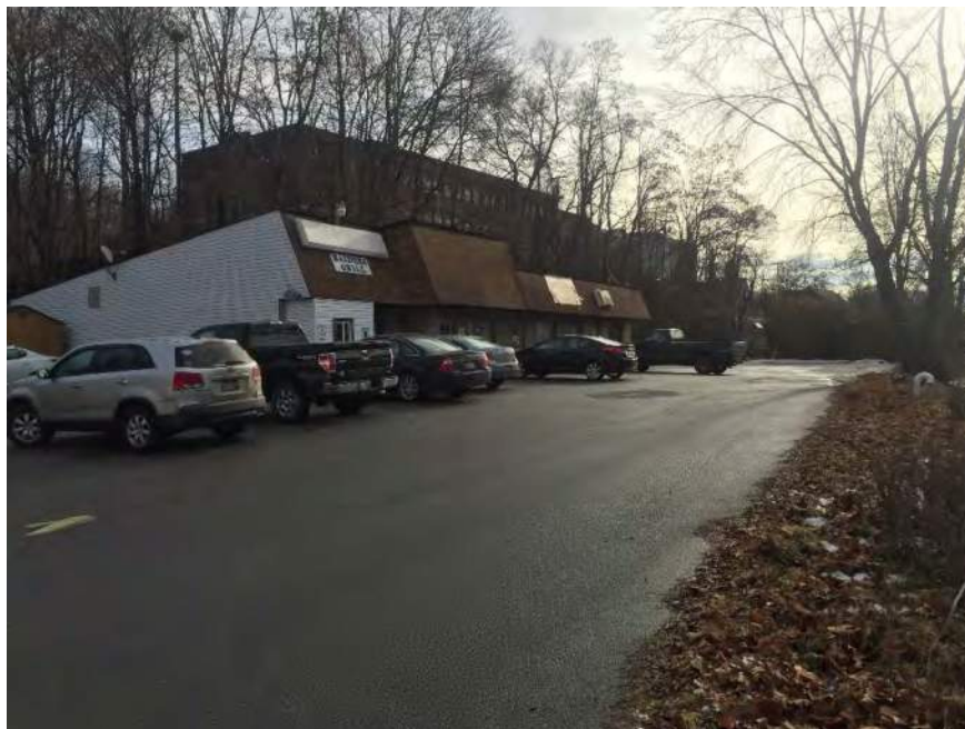
Photograph 12: View facing southeast along Raiders Grill shops. Railroad tracks to the right.
