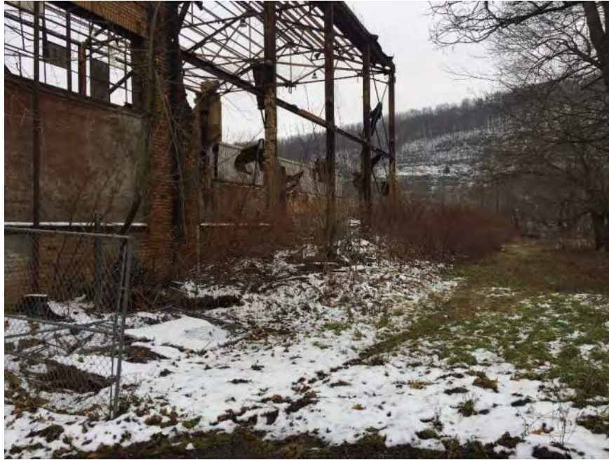
Photograph 15: View of north side of American Industrial Recycling facility.
