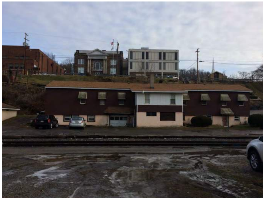
Photograph 8: View of the 212 Madison Street property (former taxi business) and the Hancock County Courthouse (background).
