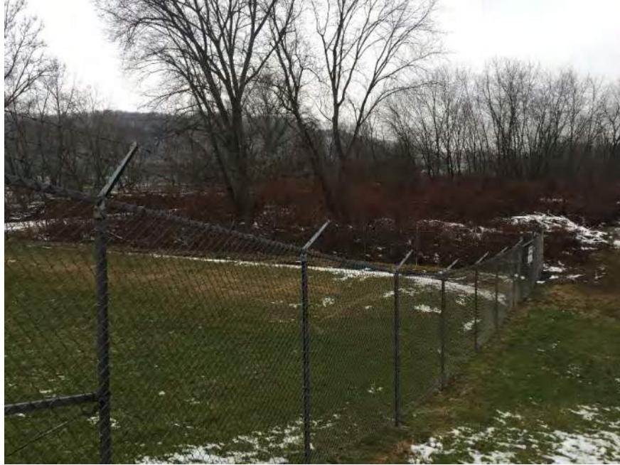
Photograph 3: Wastewater treatment plant (fenced in) and adjacent property, view looking northwest from Industrial Park Road.
