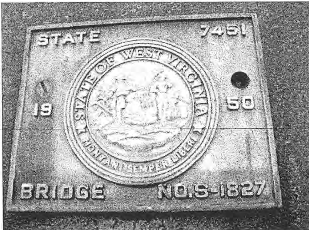
Photo #2: Bridge plate located on truss member at northern end of bridge.
