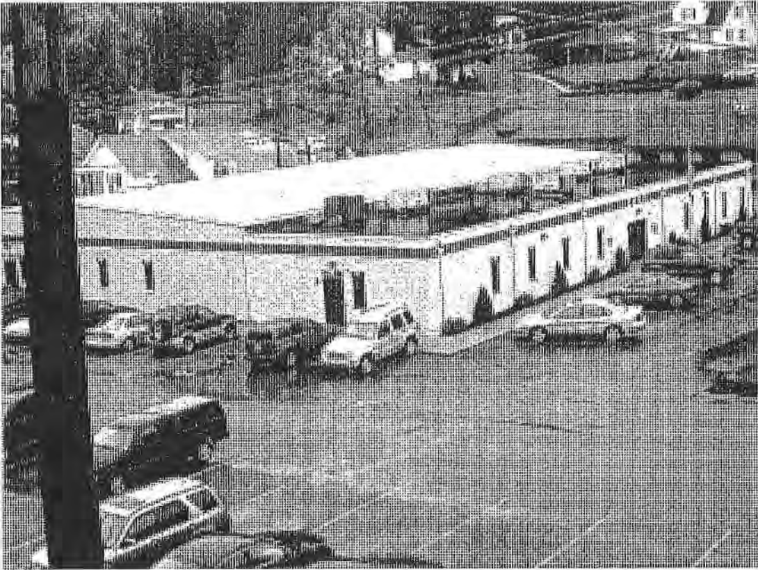
Photo #13: Looking at DHHR building southeast of bridge.
