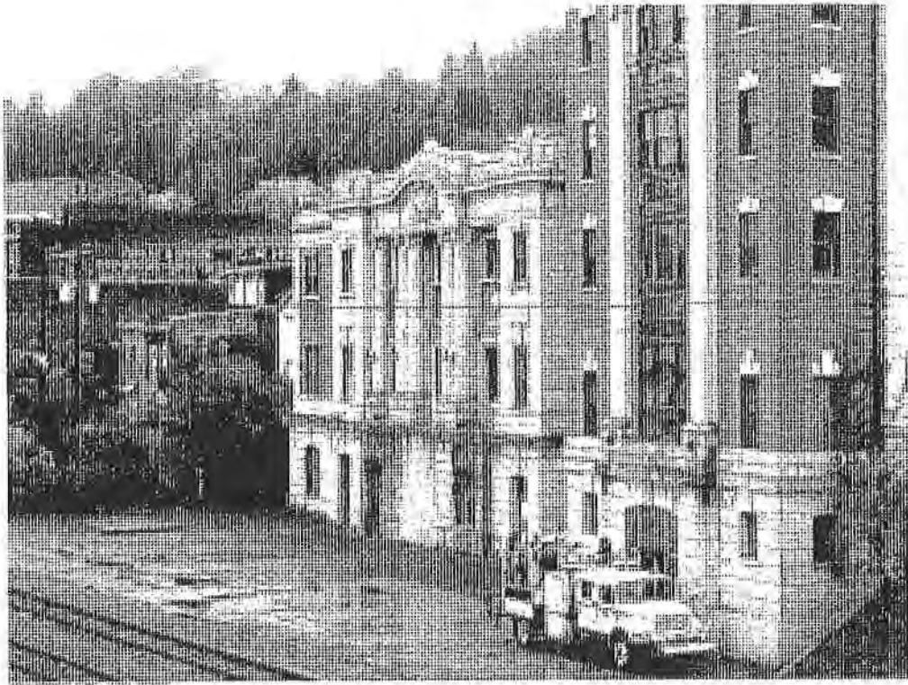
Photo #11: View of B&O depot from bridge.
