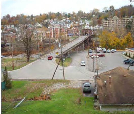
Photograph 1. The Bridge Street Bridge, Looking North.
