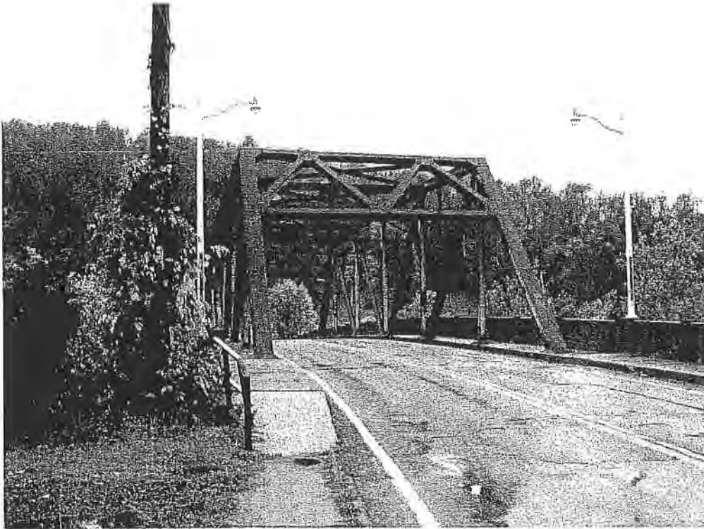
Photo #1: Bridge Street Bridge looking south at span 1, through truss.
