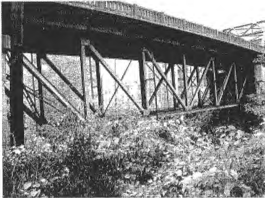
Photo #4: Looking at span 2, deck truss.
