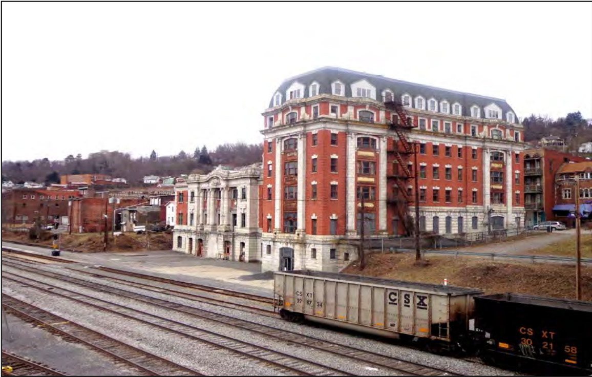
Photograph 5 – Grafton Downtown Commercial Historic District, showing Vacant Lot, Willard Hotel, and B&O Station, Facing Northwest from Bridge Street Bridge.
