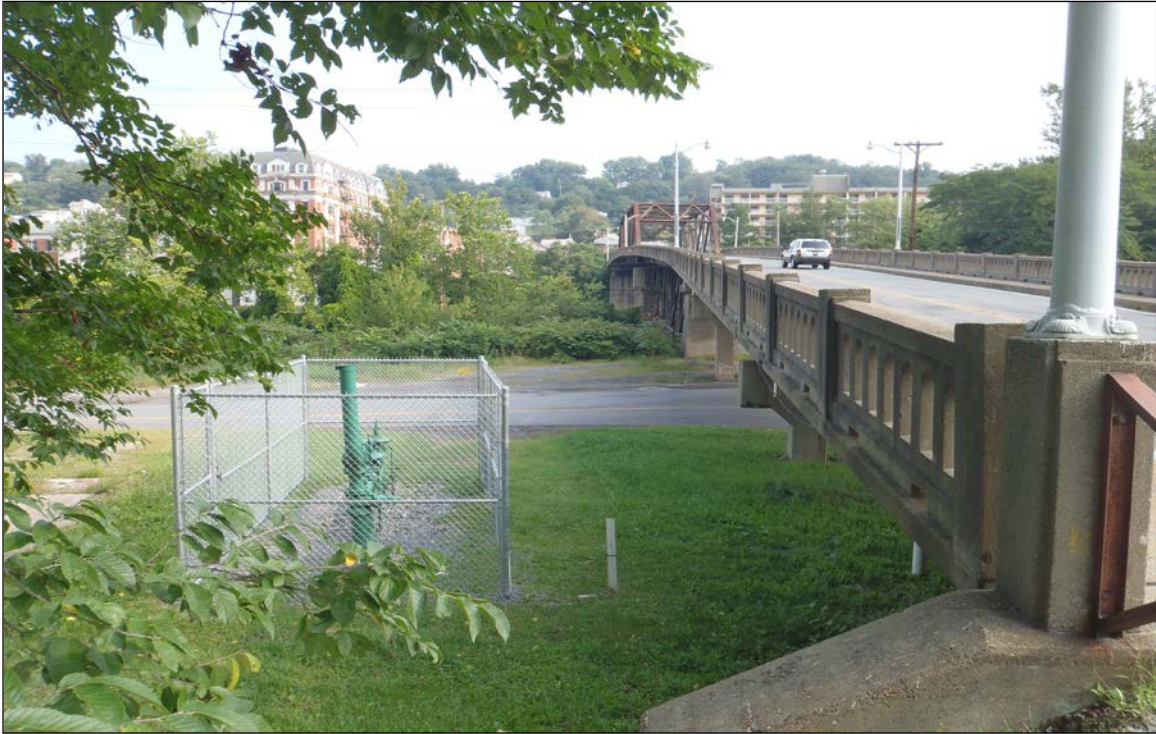
Photograph 1 – Bridge Street Bridge, Facing Northeast from South End.
