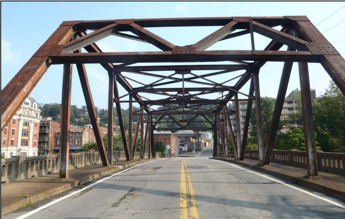
Photograph 2 – Bridge Street Bridge through Truss Facing North to Main Street.
