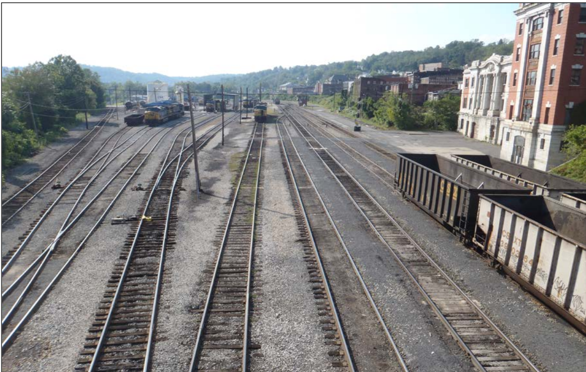
Photograph 6 – B&O Railroad and Yard, Facing West from Bridge Street Bridge.
