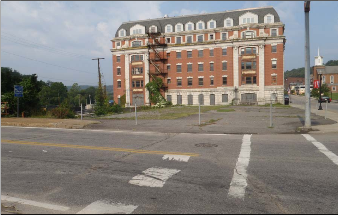
Photograph 3 – Grafton Downtown Commercial Historic District at North End of Bridge Street Bridge, showing Vacant Lot and Willard Hotel, Facing West.
