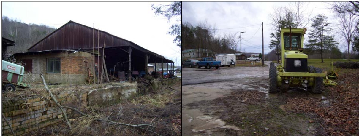
Figure 3: Portions of Coonskin Park maintenance area overlapped by Alternative 5. (Photo taken by WVDOH, 2010)
