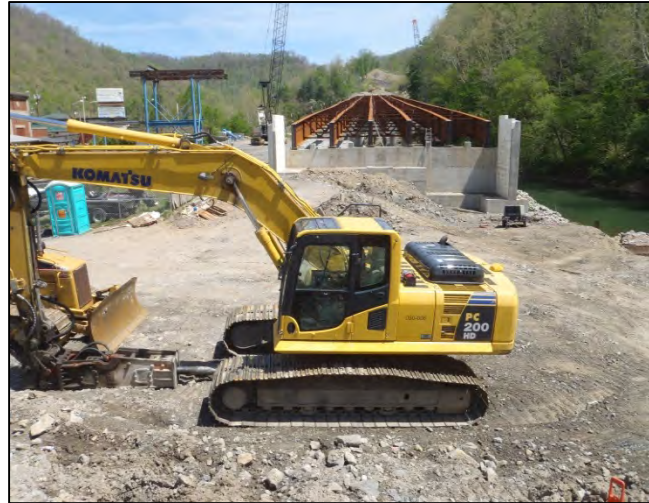
Photograph 2. WV 10 Upgrade (4-27-14), Starting at Southern End of Logan Boulevard
