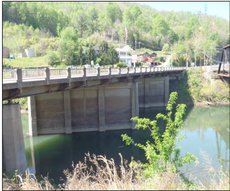
Photograph 1. Dingess Street Bridge, Looking West
