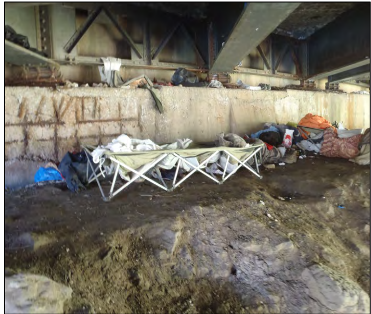
Photograph 3. Homeless Use of East End of Bridge
