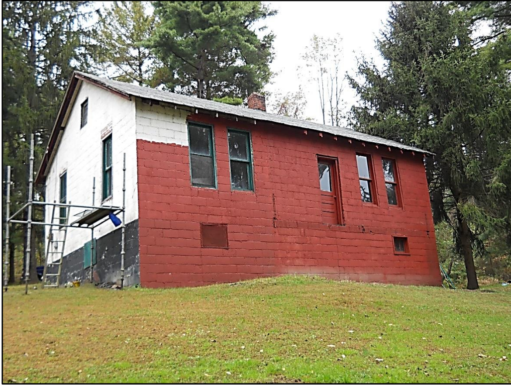
Photograph of the rear of AL-1, looking northeast.
