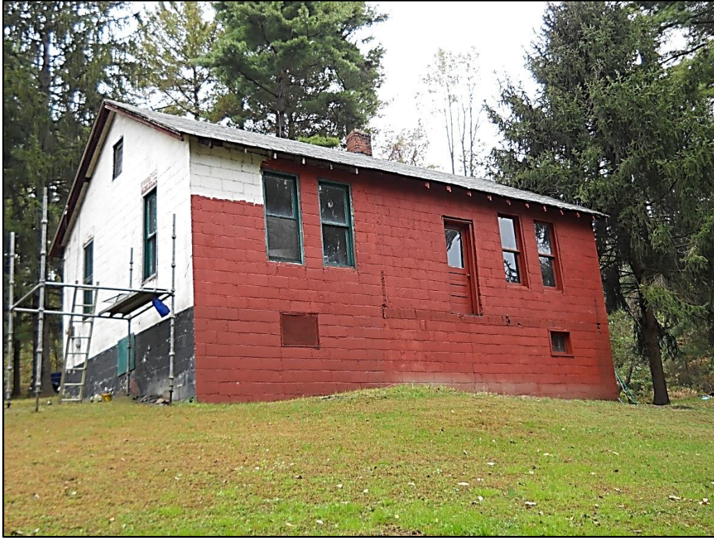
Plate 7. Photograph of the rear of AL-1, looking northeast.
