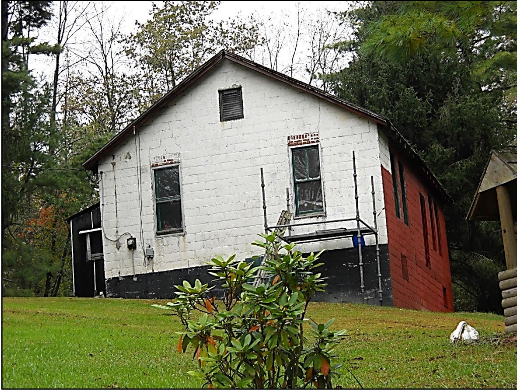
Plate 5. Photograph of AL-1 showing the brick above the windows and the addition, looking east-northeast.
