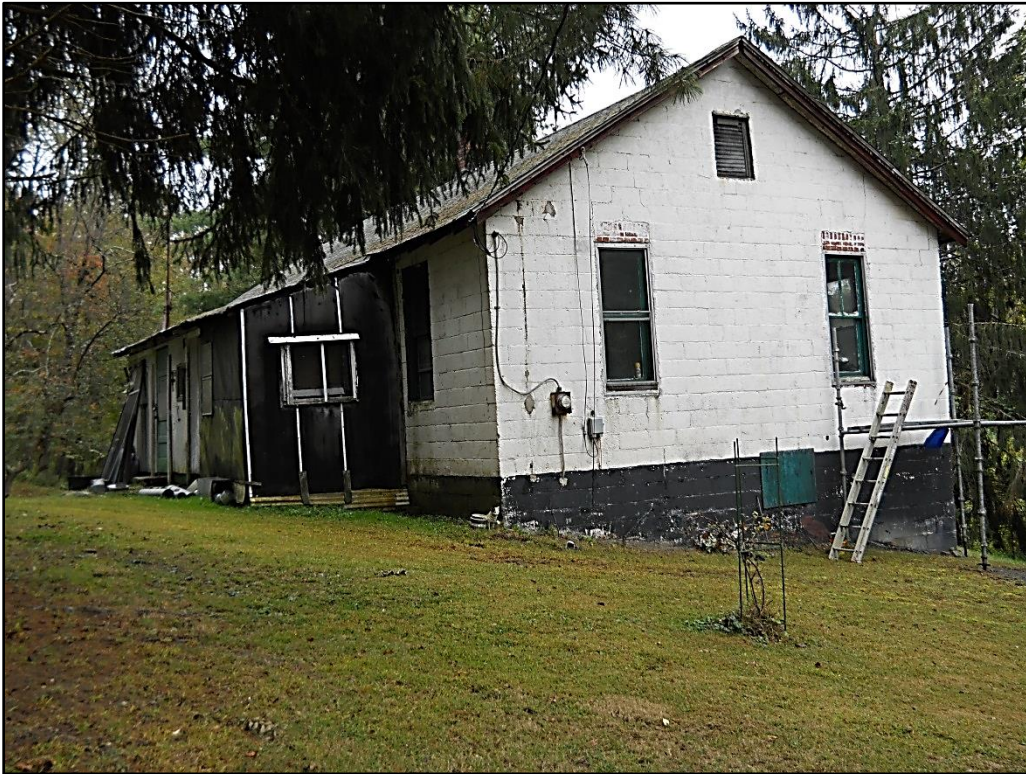
Photograph of the front of AL-1 showing the addition, looking east-southeast.
