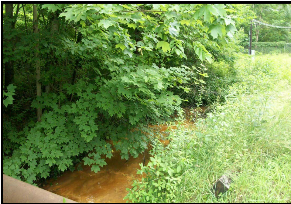
Photo #18 View of AMD treatment ditch on Consol Property.
