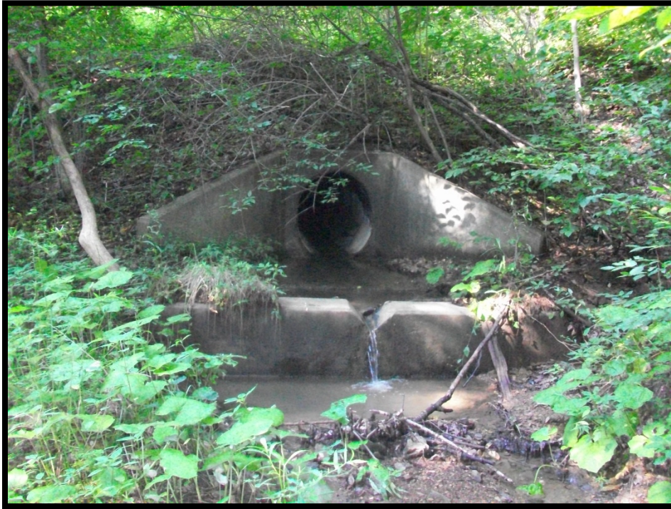
Photo #11 Stream 5 culvert under I-79.
