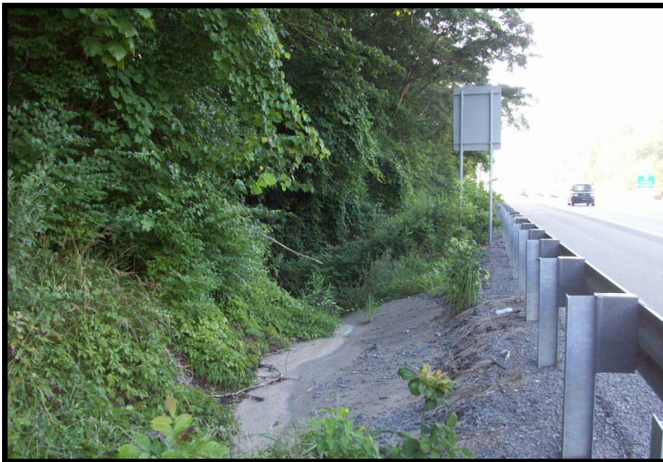
Photo #14 Typical concrete gutter along I-79 in study area.
