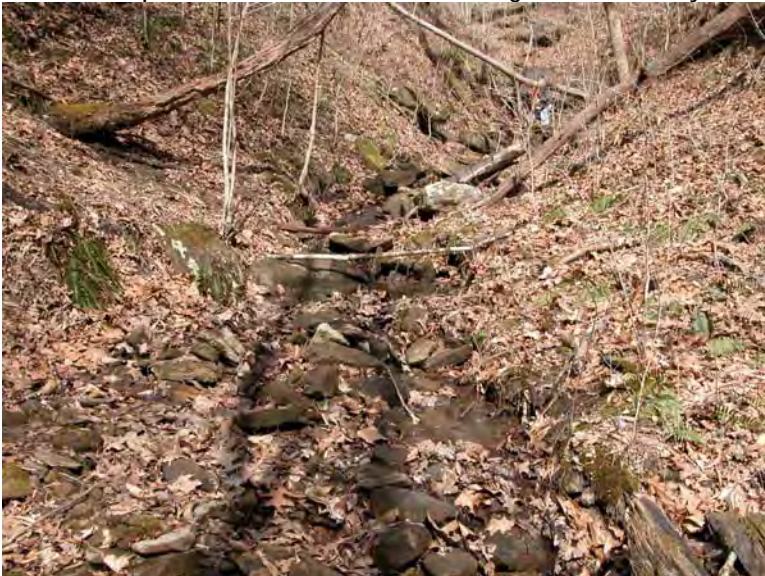
Photos 96: Proposed Restoration for Pond 2 on UT3 of Right Fork of Conley Branch
