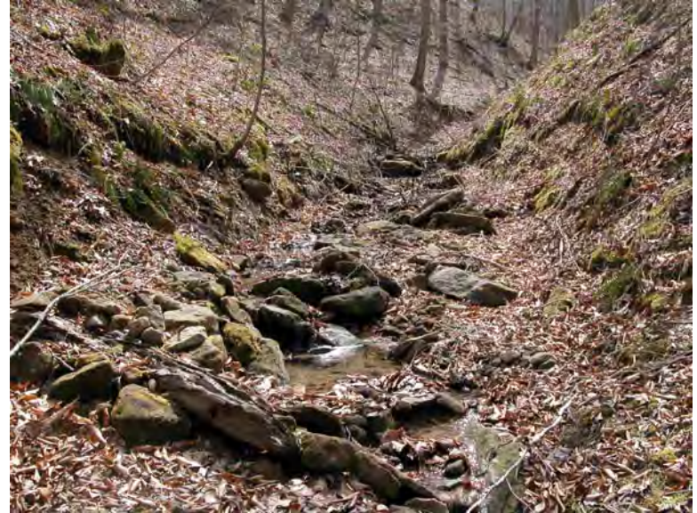
Photos 95: Proposed Restoration for Pond 2 on UT2 of Right Fork of Conley Branch
