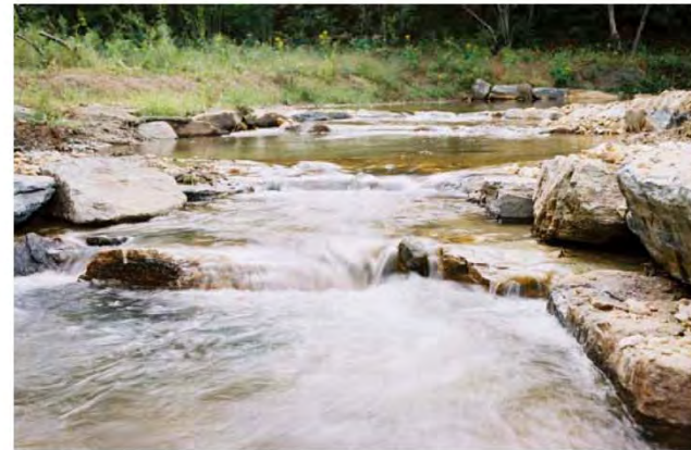
Double Drop Rock Cross Vane
