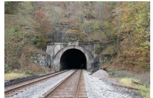
Graham Tunnel North Portal
