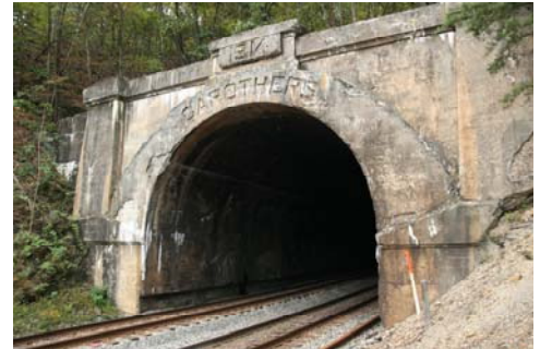
Carothers Tunnel East Portal
