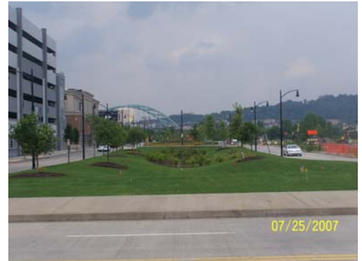
J&L Tunnel Open Space Area
