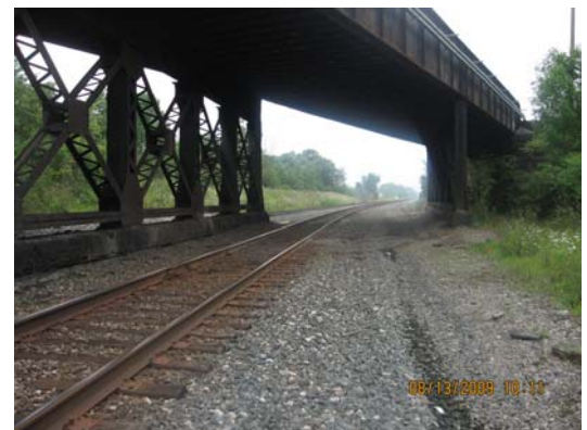
NS Railroad Bridge Ravenna Track Lowering Grade Adjustment
