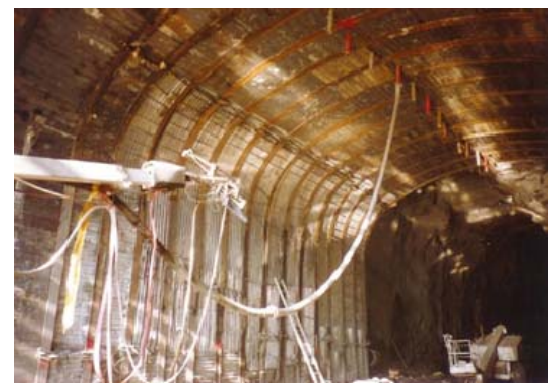
Total Arch Liner Replacement
