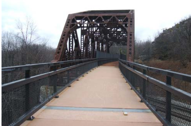
Blue Lick Truss Trail Entrance
