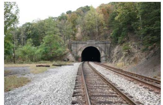
Randolph Tunnel West Portal
