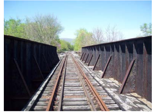
Mexico Farms Railroad Bridge Removal
