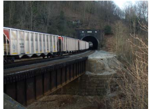
Falls Cut Tunnel
