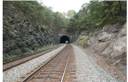
Stuart Tunnel East Portal
