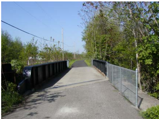
Kent Hike and Bike Trail Bridge Raising
