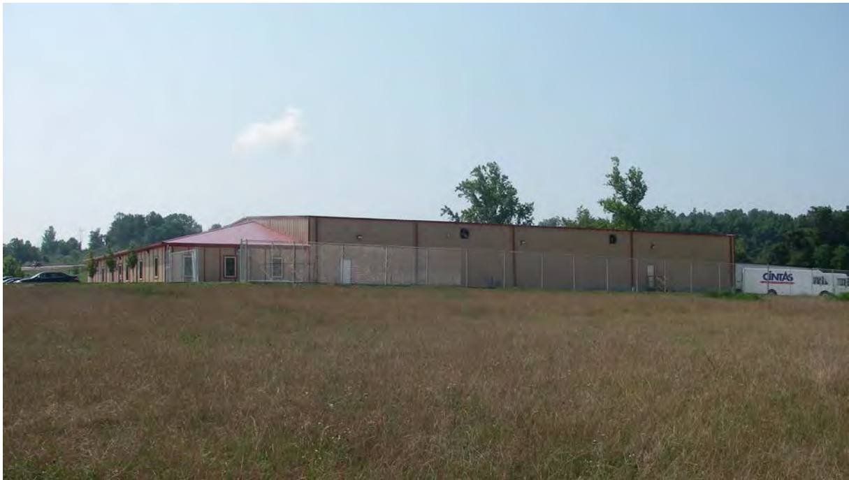
Figure 2. New Cintas business facility at southern end of project. Top: View from across WV 14 sent by WVDOH District 3 Office at beginning of EA comment period. Bottom: View from the back of the new Cintas building; WV 14 is visible in the far left background.
