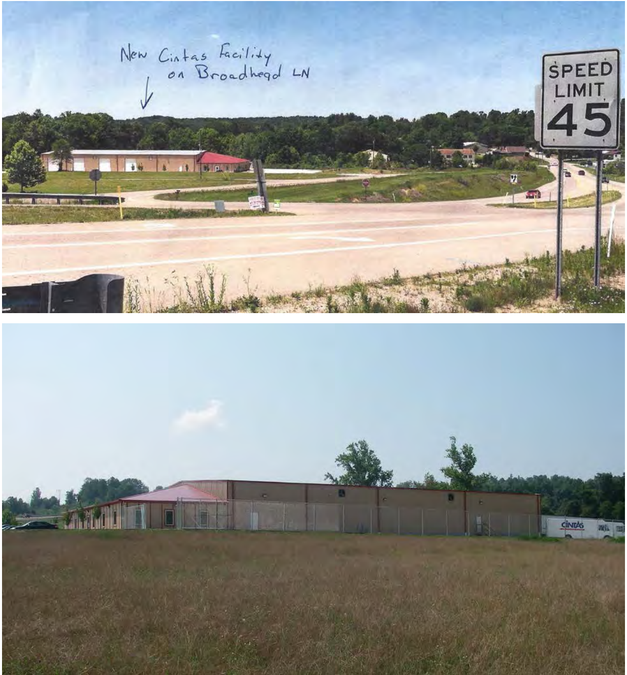
Figure 1. New Cintas business facility at southern end of project. Top: View from across WV 14 sent by WVDOH District 3 Office at beginning of EA comment period. Bottom: View from the back of the new Cintas building; WV 14 is visible in the far left background.
