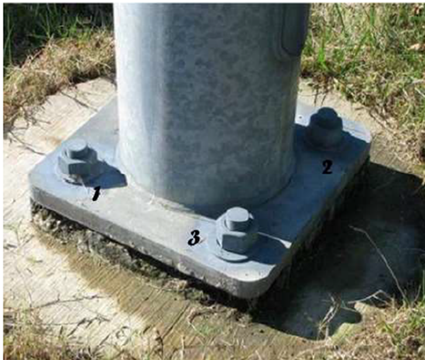
FIGURE 2 -SNUG TIGHTENING SEQUENCE NUMBERING ON BASE PLATE
