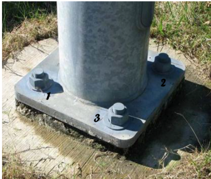
FIGURE 2 -SNUG TIGHTENING SEQUENCE NUMBERING ON BASE PLATE
