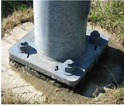
SNUG TIGHTENING SEQUENCE NUMBERING ON BASE PLATE
