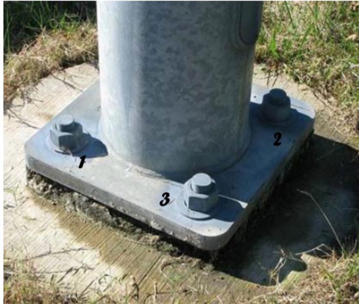
FIGURE 2 -SNUG TIGHTENING SEQUENCE NUMBERING ON BASE PLATE
