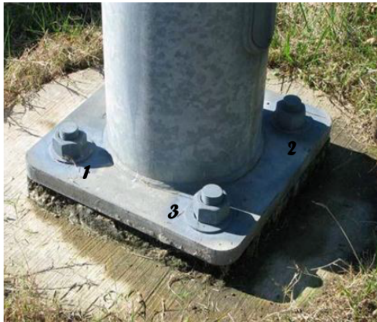
FIGURE 2 -SNUG TIGHTENING SEQUENCE NUMBERING ON BASE PLATE
