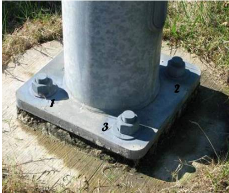
FIGURE 2 -SNUG TIGHTENING SEQUENCE NUMBERING ON BASE PLATE
